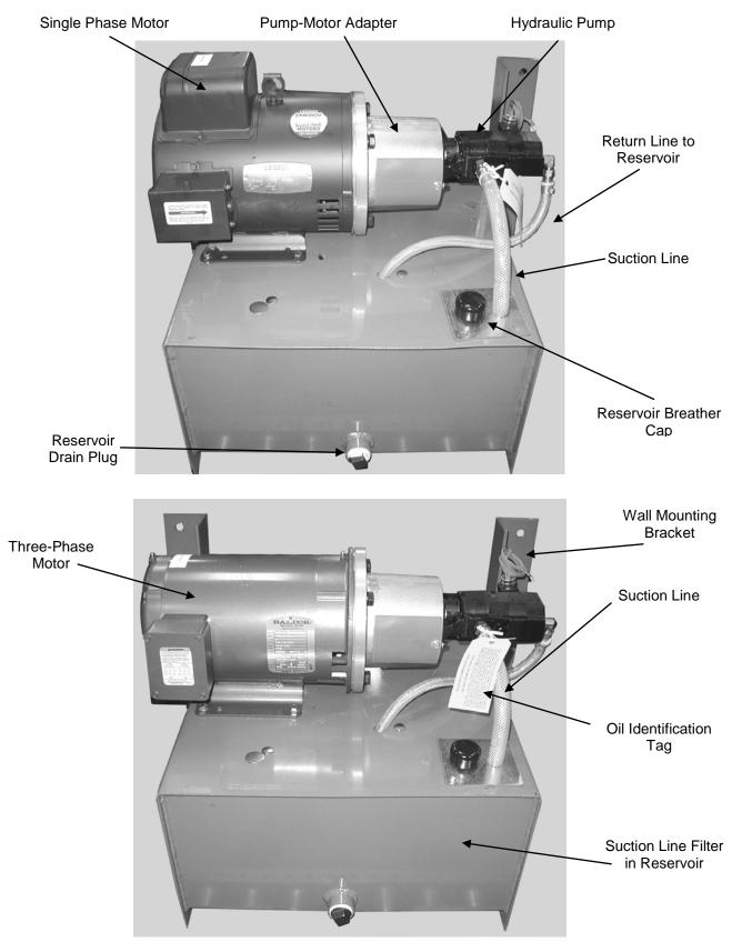
See Page 8-4 for Hydraulic Diagram and Pages 9-3 thru 9-5 for Electrical Diagram
